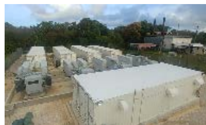
Talofofo BESS 16 MW Frequency Regulation
