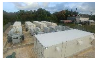
Talofoto BESS 16 MW Frequency Regulation
