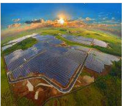
Dandan Solar 25 MW – Ph I
